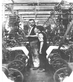
FACTORY WORKERS SOURCE: PPTP/WWW.LEARNINGMUSE.COM
